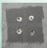
5. Mask the grounding plate, but do not overpaint it! Overpaint the area with commercial wall paints, wallpapers or use fine plaster as recommended in the corresponding technical data sheets.
